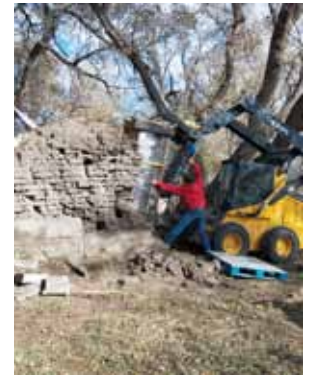
Using rope, pallets, and a forklift, volunteers carefully lay the sod wall down.
