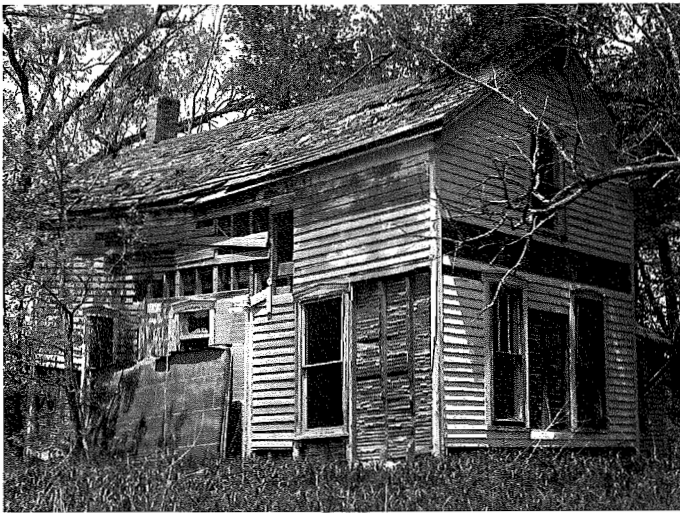
Fig. 8a. Mixed building techniques made a sagging, unstable structure of this one-and-a-half story farmhouse in Otoe County, Nebraska (c.1880). Framed with 4" by 4" corner posts and 2" by 4" wall studs, it lacks external sheathing and is supported on only eight brick piers. Courtesy the author
