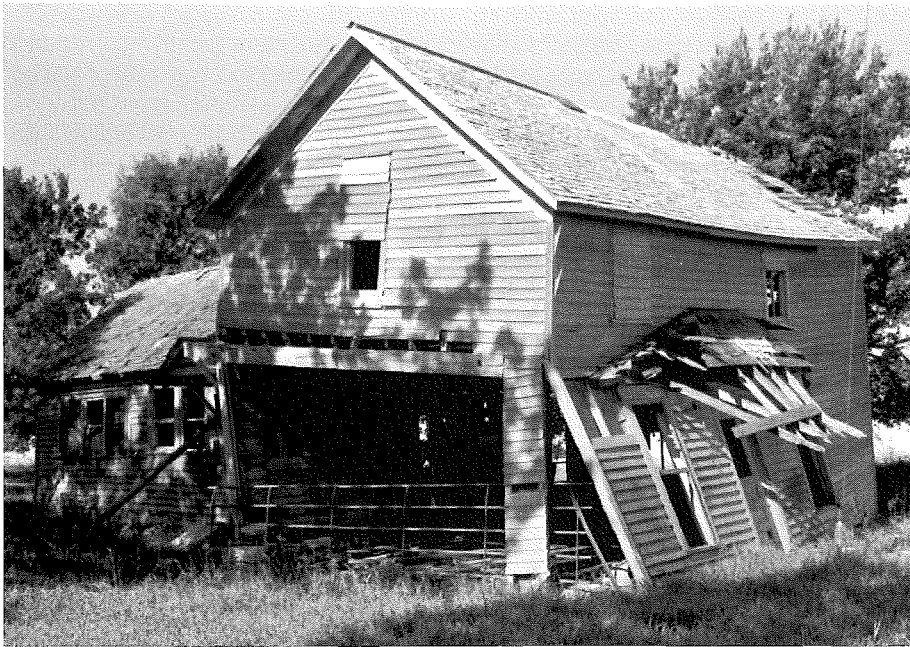
Fig. 7. The builder of this farmhouse in Pawnee County, Nebraska (c.1870), apparently did not fully understand milled-lumber-and-nail construction; instead of running studs continuously from sill to plate, he built the first story as a platform for the half story above it. Winter winds buckled it at the junction. Courtesy the author
