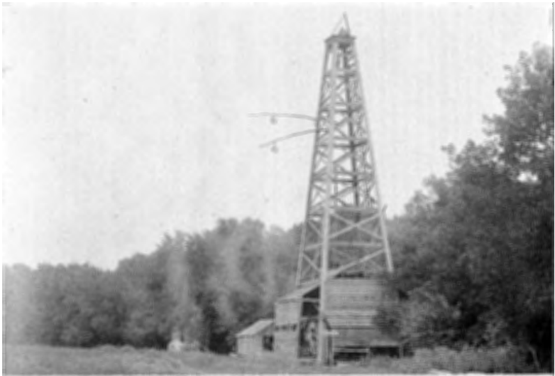
Oil derrick on the Morris farm near Shelton, Buffalo County, in 1910.
