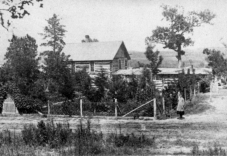
Above: Mead's Tavern and home, south bank of the Niobrara River, about 1886.
