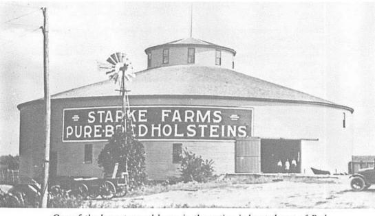
One of the largest round barns in the nation is located east of Red Cloud, Webster County. Built in 1902-1903 by the Starke brothers, the structure features a central silo 28 feet in diameter and 65 feet high. The interior, composed of three levels, is 130 feet in diameter.
