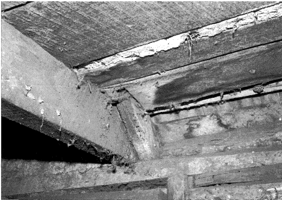
Fig.12. Veselý house, Knox County. Interior view showing the joists and rafters connecting to the lumber plate atop the plate log, the split-log filler closing the space between the roof sheathing and the plate, and the loft floorboard. Mud plaster insulation on the loft floor can be seen between the floorboards. D. Murphy, NSHS RG1763-8212/4:12
