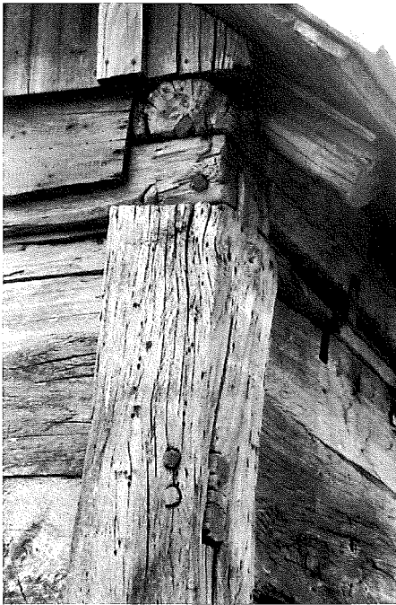
Fig. 5. Corner detail of the post-and-panel construction of the Skala house, now at Battle Creek, showing the connections at the plate. D. Murphy, NSHS RG1763-7908/3:7
