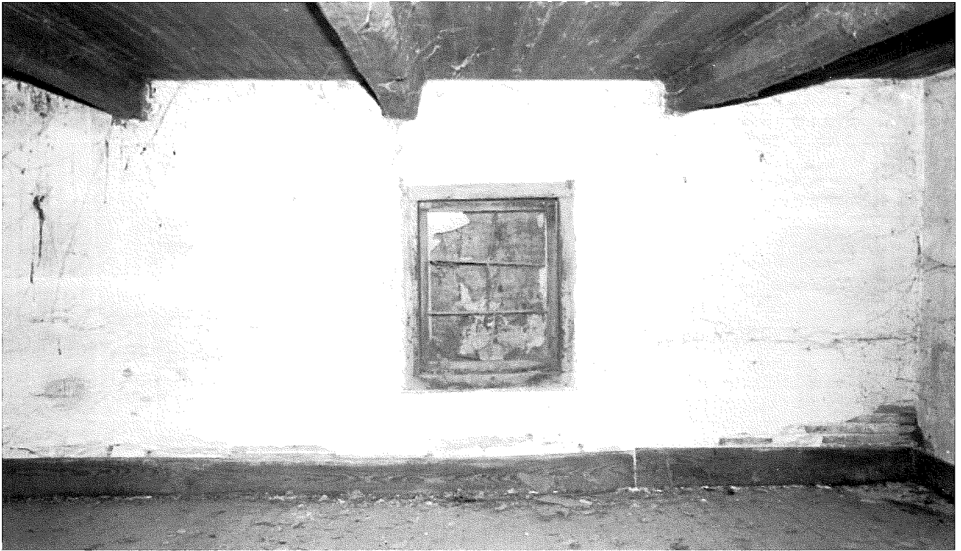
Fig. 24. Interior view of the main room of the Eckstein-Buresh house, Saunders County, showing the chamfered tie beams, board ceiling, and lath and plaster wall finish. D. Murphy, NSHS RG1763-8008/23:9
