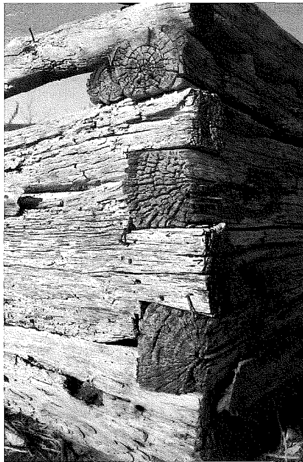
Fig. 6. Detail of the corner timbering of the hewn timber crib of the Mářšl double-crib barn, Knox County, showing the slightly splayed full-dovetail notches. D. Murphy, 8511-5
