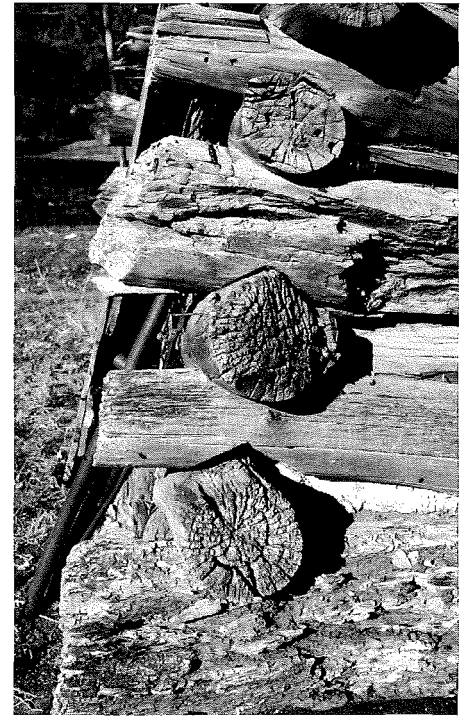
Fig. 19. Detail of the V-notched corner timbering in the Kounovský smokehouse, Knox County. D. Murphy.
