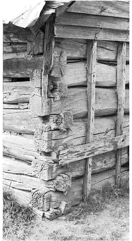
Fig. 16. Detail of the vertical double-notch corner timbering in the Veselý house. D. Murphy, NSHS RG1763-8010/7:1
