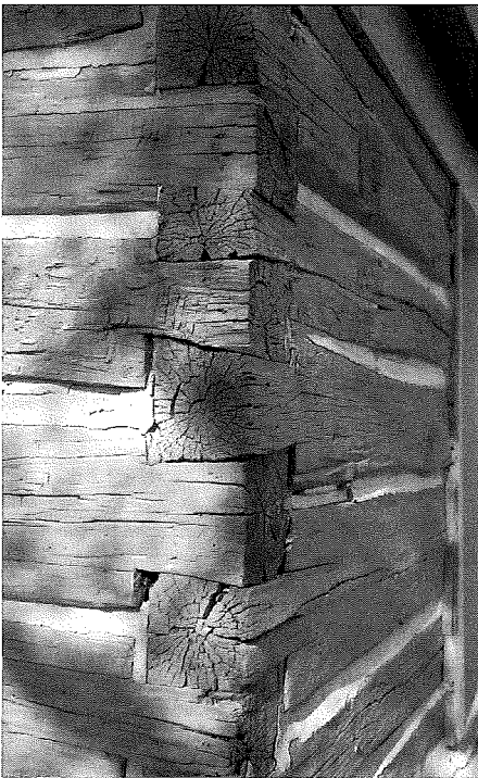
Fig. 17. Detail of the half-dovetail variants in the full-dovetail corner timbering of the Tabor School, Tabor, South Dakota. D. Murphy, 8511-11
