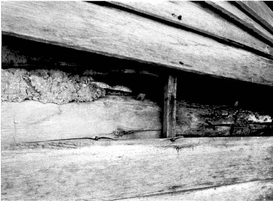
Fig. 8. Detail of the chinking in the Šrajer-Dryák house, Pischel Creek, showing the shape of the logs, the remnant clay and wood chinking, and the wedge-shaped pegs used to “lath” the clay in place. The view is through a gap in the siding, and shows a furring strip. D. Murphy, NSHS RG1763-8804/2:4
