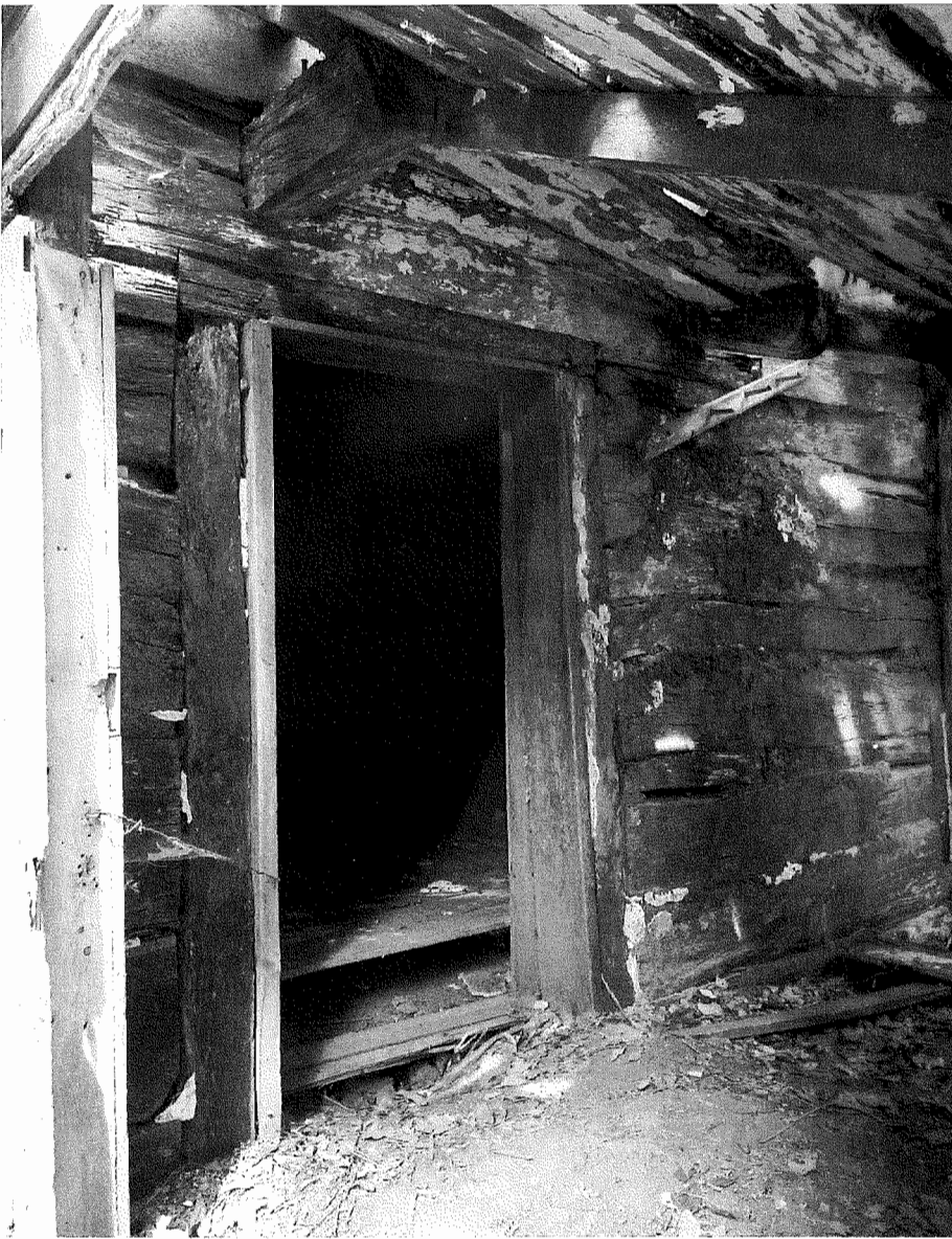
Fig. 10. Ekstein-Buresh house, Saunders County. View of the main entrance inside the mud porch showing the mortised-post door frame and the protruding tie beams. The common rafter for the main roof can be seen connecting into the top of the nearest beam at the top of the photograph, while the rafters for the shed-roofed mud porch are spiked to the side of the beams. Remnants of mud plastering and whitewash are also visible. D. Murphy, 8008-2
