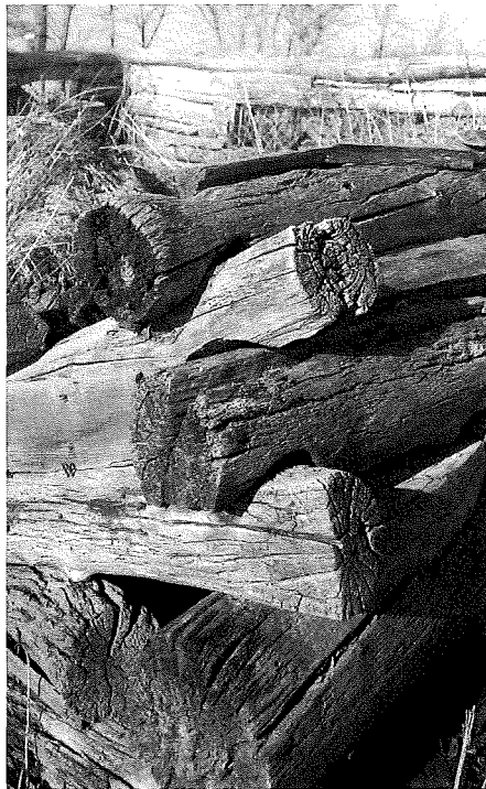
Fig. 18. Detail of the saddle-notched corner timbering in the unhewn crib of the Mářšl double-crib barn, Knox County. D. Murphy, 8511-6
