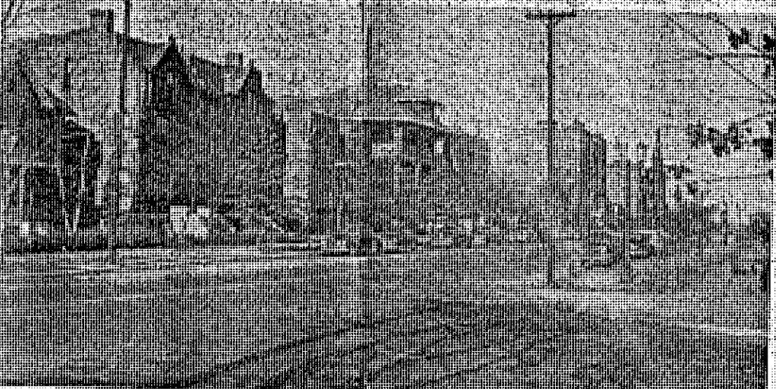
Best section of the building's structure is in the west, along Fourteenth Street, where these apartments are located.
