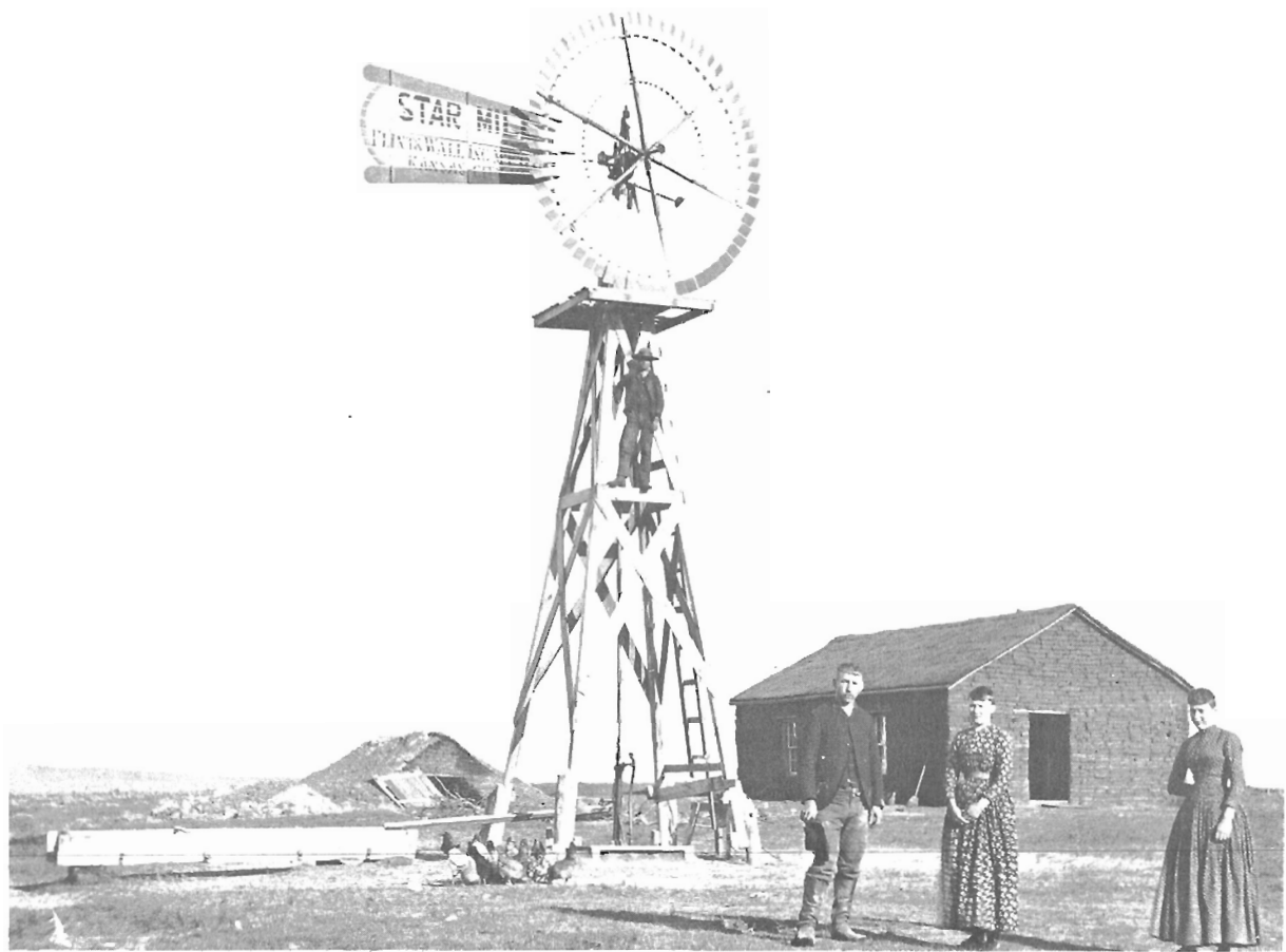
Flint & Walling manufactured the Star mill featuring a solid-type wheel. In this farm scene from Custer County (ca. 1887), notice the new sod house, the boy on the windmill platform, and the cluster of chickens at its base. (Photo, S. D. Butcher collection)
