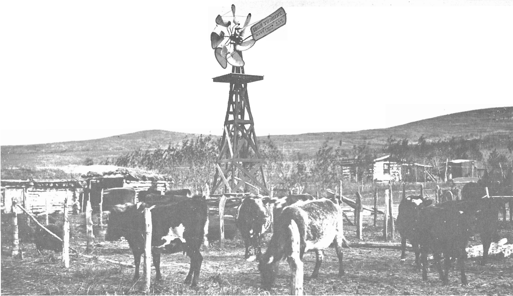
The "Iron Turbine" had the first all-metal windmill head. About 1886 this homestead in Custer County was owned by T. Cozad. The shed and house in the background are of log construction. (Photo, S. D. Butcher collection)
