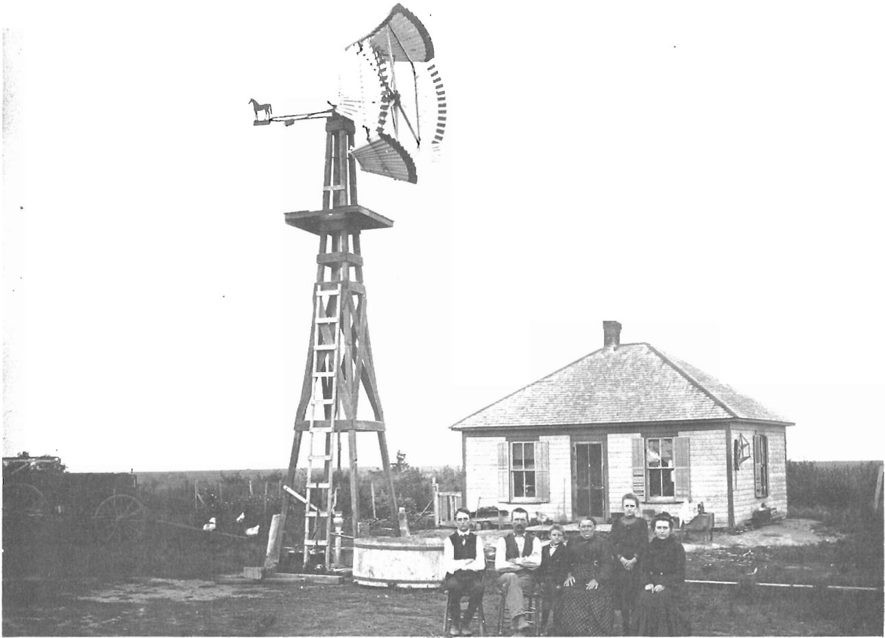
Note the “horse” counterweight on the Dempster “vaneless” type windmill. The wheel is shown in the folded or furled position. Mike Sturm and family lived on this farm near Kearney, Buffalo County. (Photo, S. D. Butcher collection)
