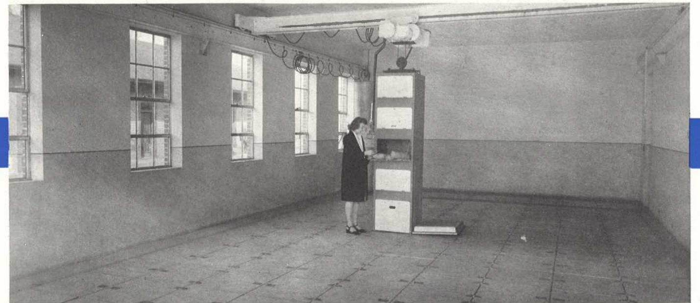
Slayton has a new and different type of freezer-locker plant. Lockers are under the floor. The renter opens the proper hatch and uses the hoist, as shown here, raising the tier in which the locker is contained.
