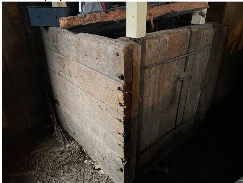
Figure 14: original water tank used to cool four 10 gallon milk jugs using well water. The tank emptied into the water trough when full.
