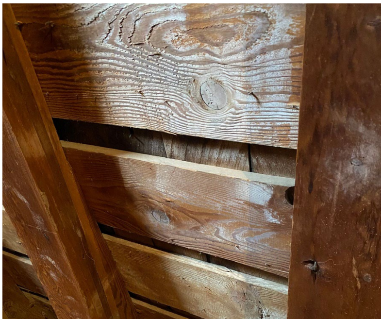
Figure 18: View of the roof decking spaced several inches apart to allow the original wood shingles (visible behind) to dry out. Also visible is the white cement remnants on some of the decking from the first use to frame in the barn foundation.
