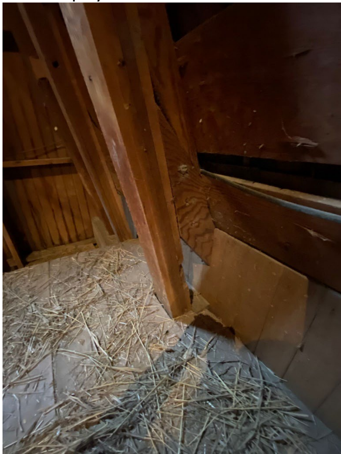
Figure 17: View of the main truss as it punches through the floor and the support flaring out to hold up the roof eave.
