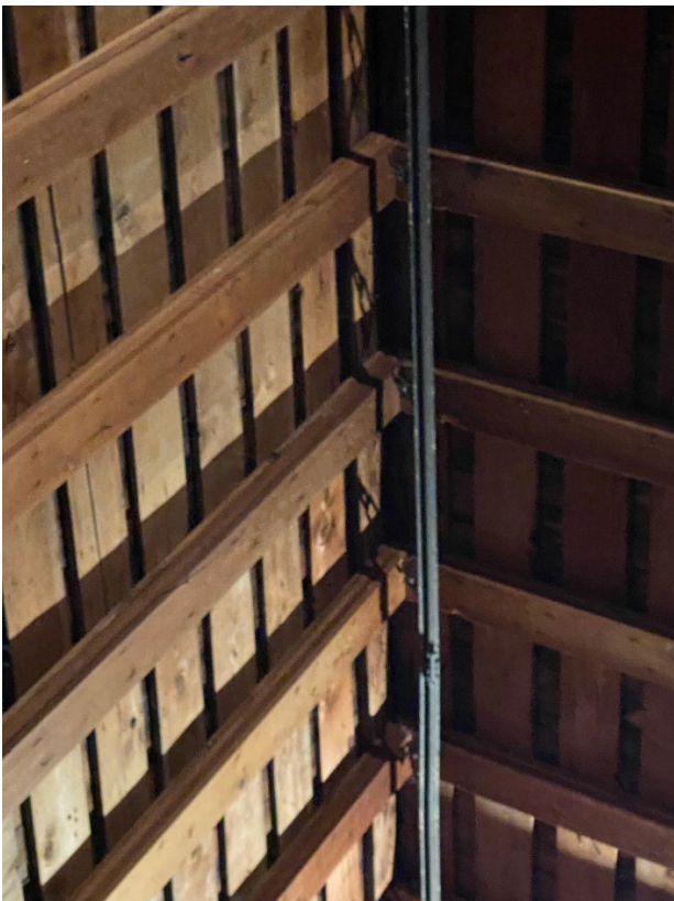
Figure 23: roof peak where the rafters meet.
