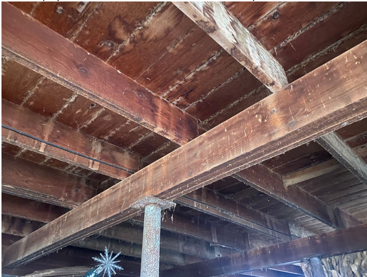
Figure 9: support structure for hayloft showing beams of three 1x12s laminated together
