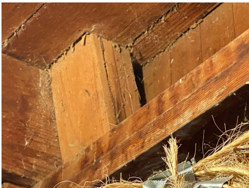
Figure 10: view of the four laminated boards comprising the roof truss projecting down to the first floor sill plate
