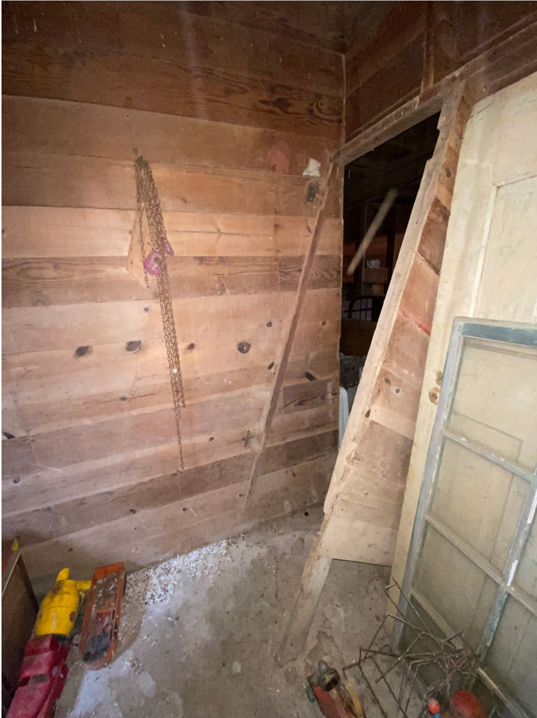
Figure 13: one of two grain rooms with angled doorway that stopped a few feet above the ground (missing doors) that allowed grain to fill the room and be scooped out from the bottom without spilling into the rest of the barn. When the area at the door was cleared, the angled door could be opened providing access to the rest of the grain in the room.
