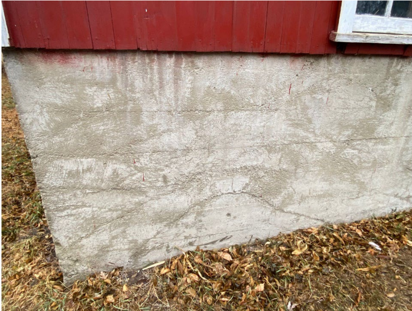
Figure 4: The waves in the poured concrete reflect the manual way in which individual wheel barrels of hand mixed concrete were poured into the molds a few at a time, allowing for the wave pattern to form.
