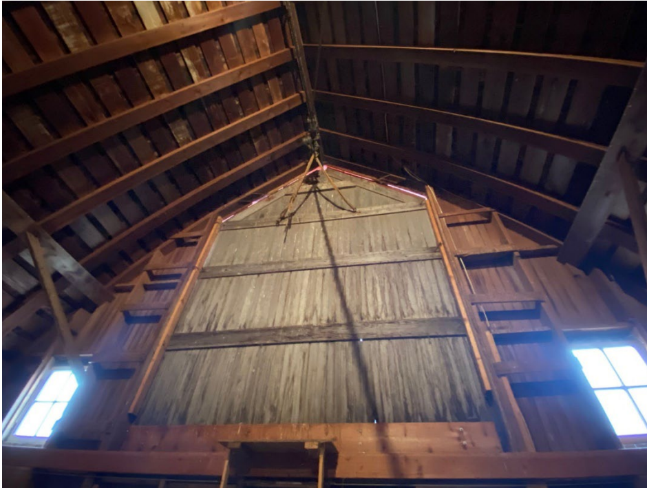
Figure 20: Interior of the large hay door, discolored from remaining open during the summers. Also visible is the pulley system at the top used to pull loose hay, then bales of hay into the loft. On either side of the door are wall ladders used to get to the door latches.
