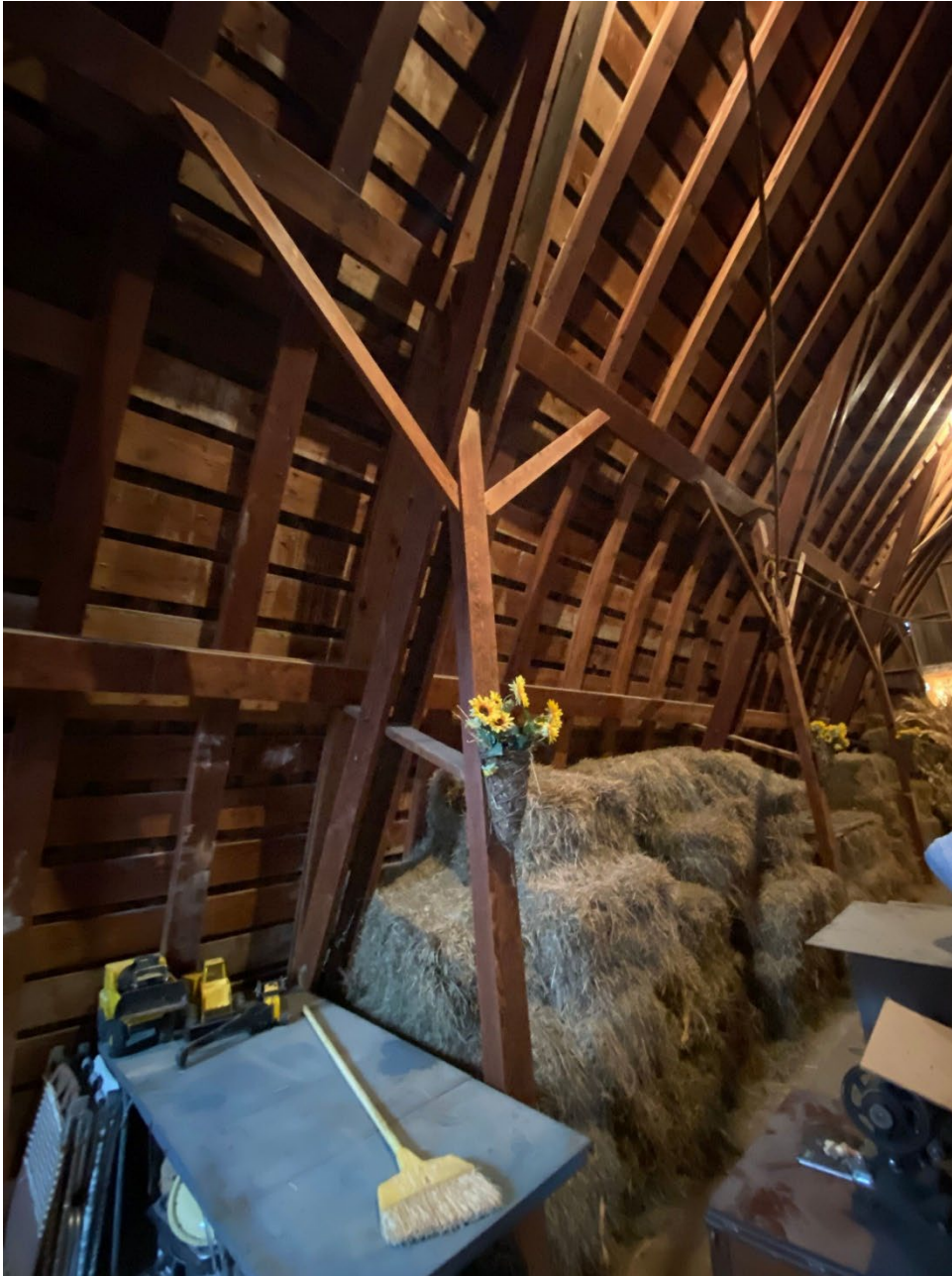
Figure 19: Y shaped supports were added in 1934 shortly after the barn was constructed to give more support since the center of the loft is completely free of columns to keep it open and easy to fill with hay.
