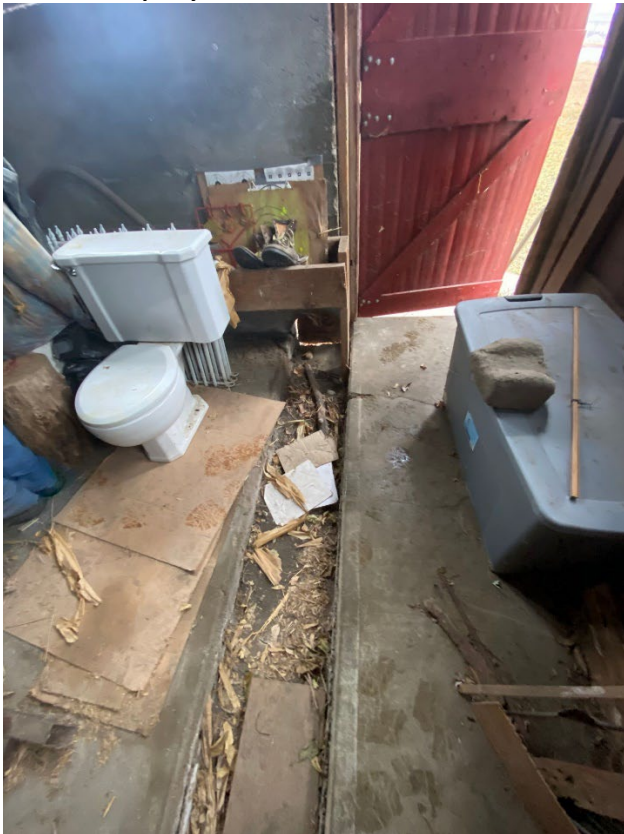
Figure 8: cement trough for washing cow excrement out of barn (center)
