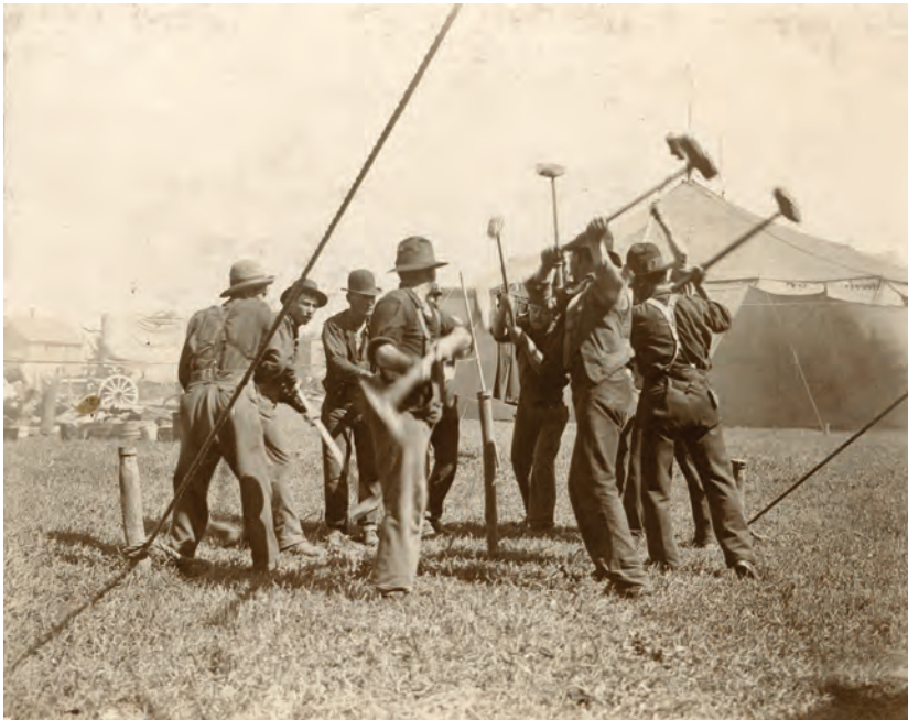
Hammer gang, Lincoln, ca. 1915. When the circus hit town, the roustabouts, canvas crews, and hammer gangs had little time to get the tents and rigging ready for the first matinee. McClure's Magazine reported in 1895 that 200-300 blows were required to drive home a five-foot tent stake. Standing in a circle, the hammer gang worked their seventeen-pound hammers with such perfect rhythm that a stake received seven blows per second, and a good crew could sink a thousand stakes in forty-five minutes. NSHS RG3322-47
