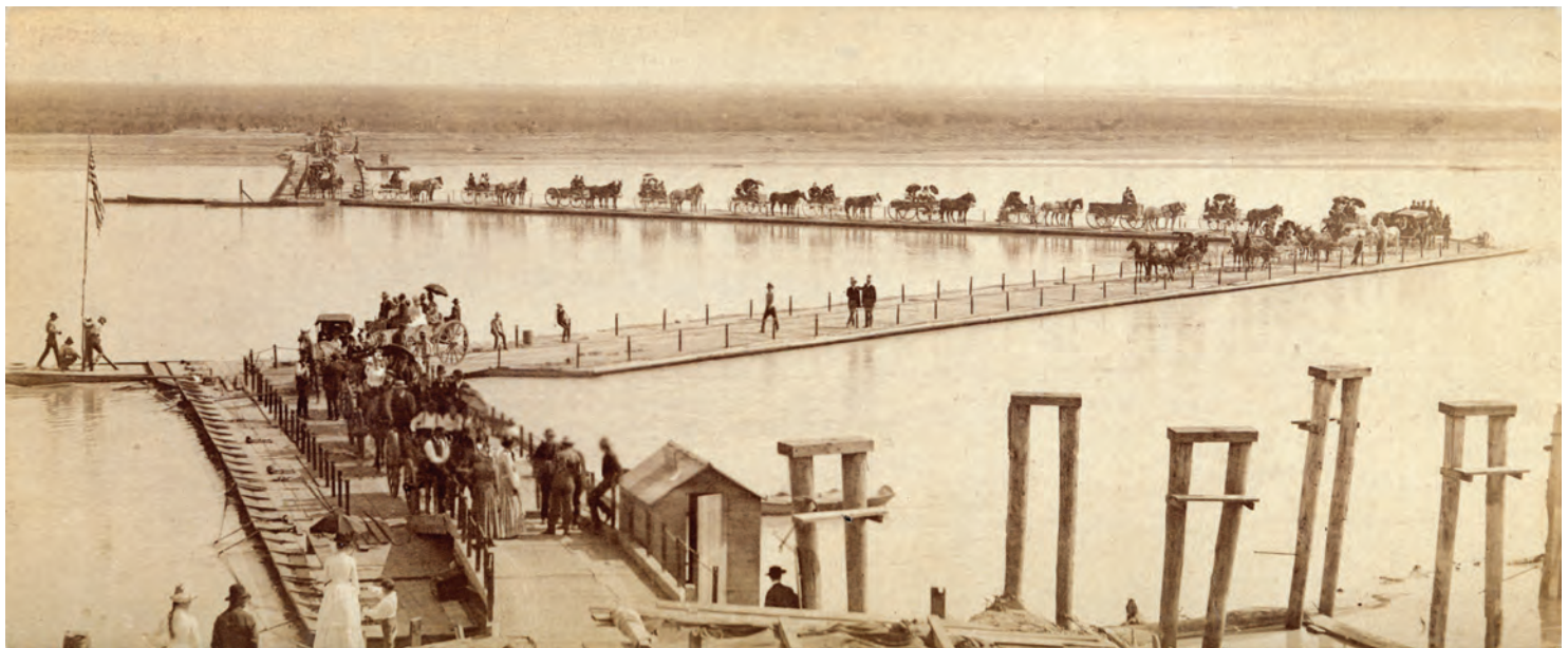
Rivers were major travel barriers for most of human history. And even after railroad bridges spanned the Missouri River, they were usually closed to wagon traffic. In 1888 Nebraska City subsidized a thousand-foot pontoon bridge, said to be the first pontoon bridge across the Missouri and the largest drawbridge of its kind in the world. The V-shaped "draw" opened for steamboats or flowing ice. The pontoon bridge served until 1891, when the Burlington Railroad added planks to its existing bridge and opened it as a toll-bridge for non-railroad traffic. NSHS RG2294-71
