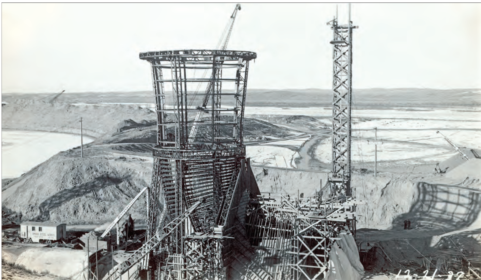
Construction of the spillway tower at Kingsley Dam, December 21, 1937. The world's second largest hydraulic-fill dam at the time of its construction, Kingsley was built by pumping sand from the riverbed, with loess clay forming the dam's watertight core. The spillway began generating electricity in 1941, and within a few years Lake C. W. McConaughy was providing irrigation water through more than 500 miles of canals and laterals. The project bears the names of two of its early promoters, George P. Kingsley, a Minden banker, and C. W. McConaughy, a grain merchant and mayor of Holdrege. NSHS RG2114-4-162
