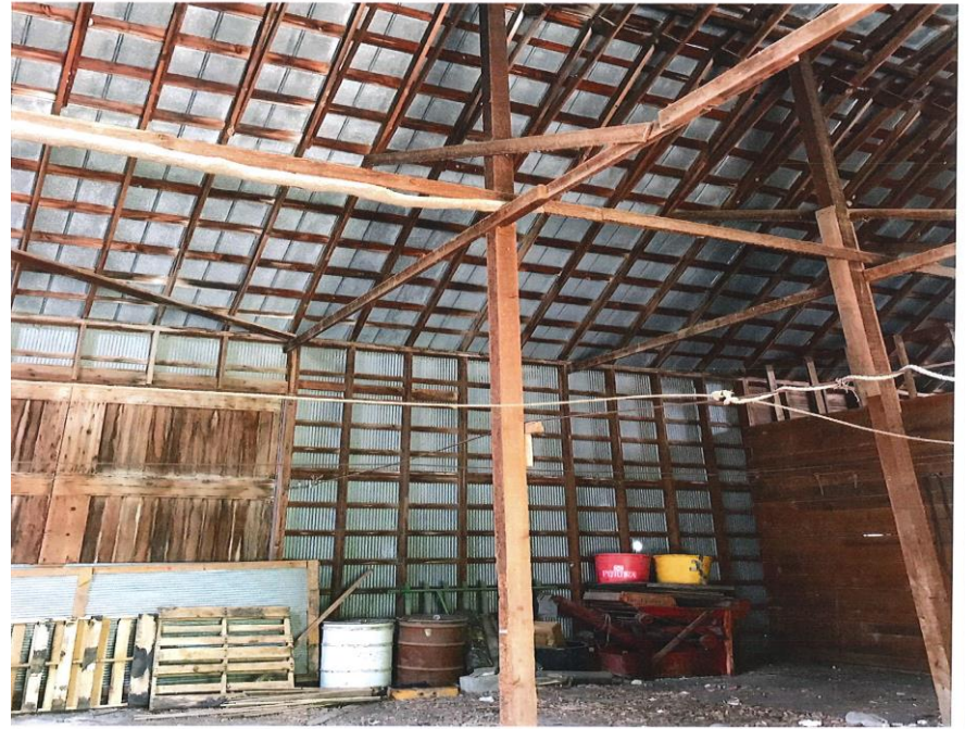
North wall and roof
