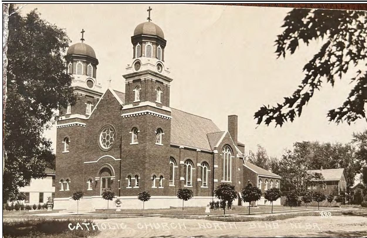
Figure 04: St. Charles Borromeo Catholic Church and Rectory with House at Right, before the mid-1930s 44
