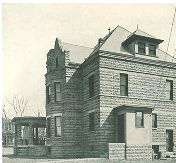
Figure 2: Photo of the northwest corner of 2060 Florence Boulevard from Tornado Proof Ambler Asbestos "Century" Shingles ; Keasbey & Mattison Company, 1917
