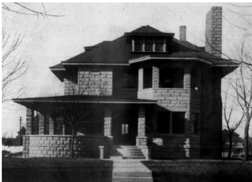
Figure 6: Photograph from Rock Products , Chicago, Illinois; February 21, 1909 of the concrete block house of Dr. R.E. Lamoreaux.
