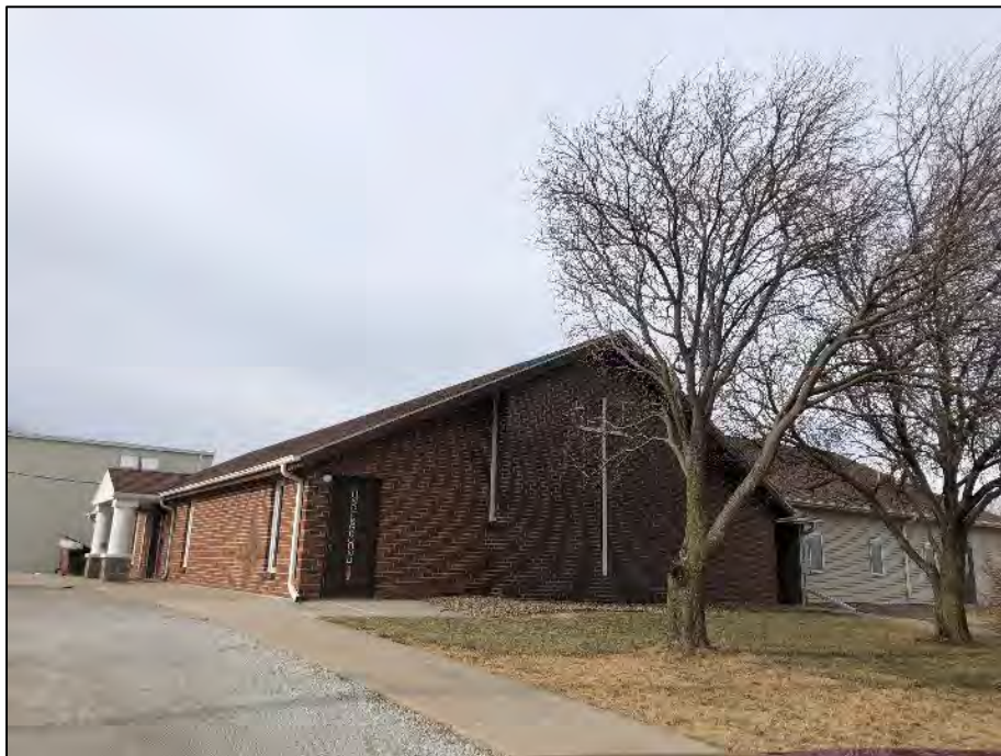
Figure 09: Evangelical Free Church, Geneva, NE, built after 1973 81
