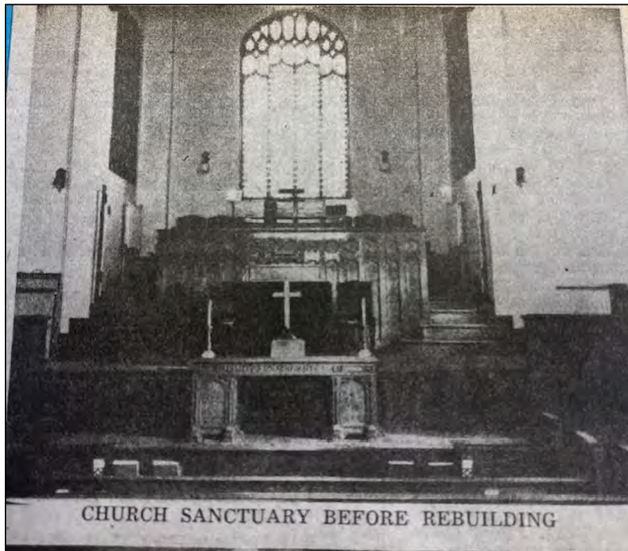
Figure 04: East end of church prior to 1967 renovation 74
