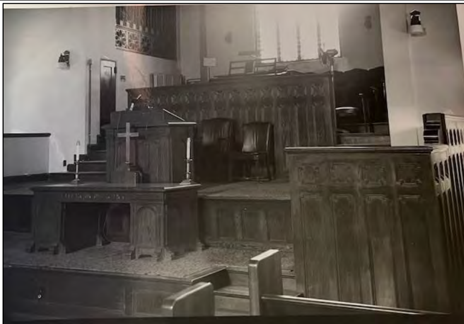
Figure 05: Chancel of church prior to 1967 renovation 75
