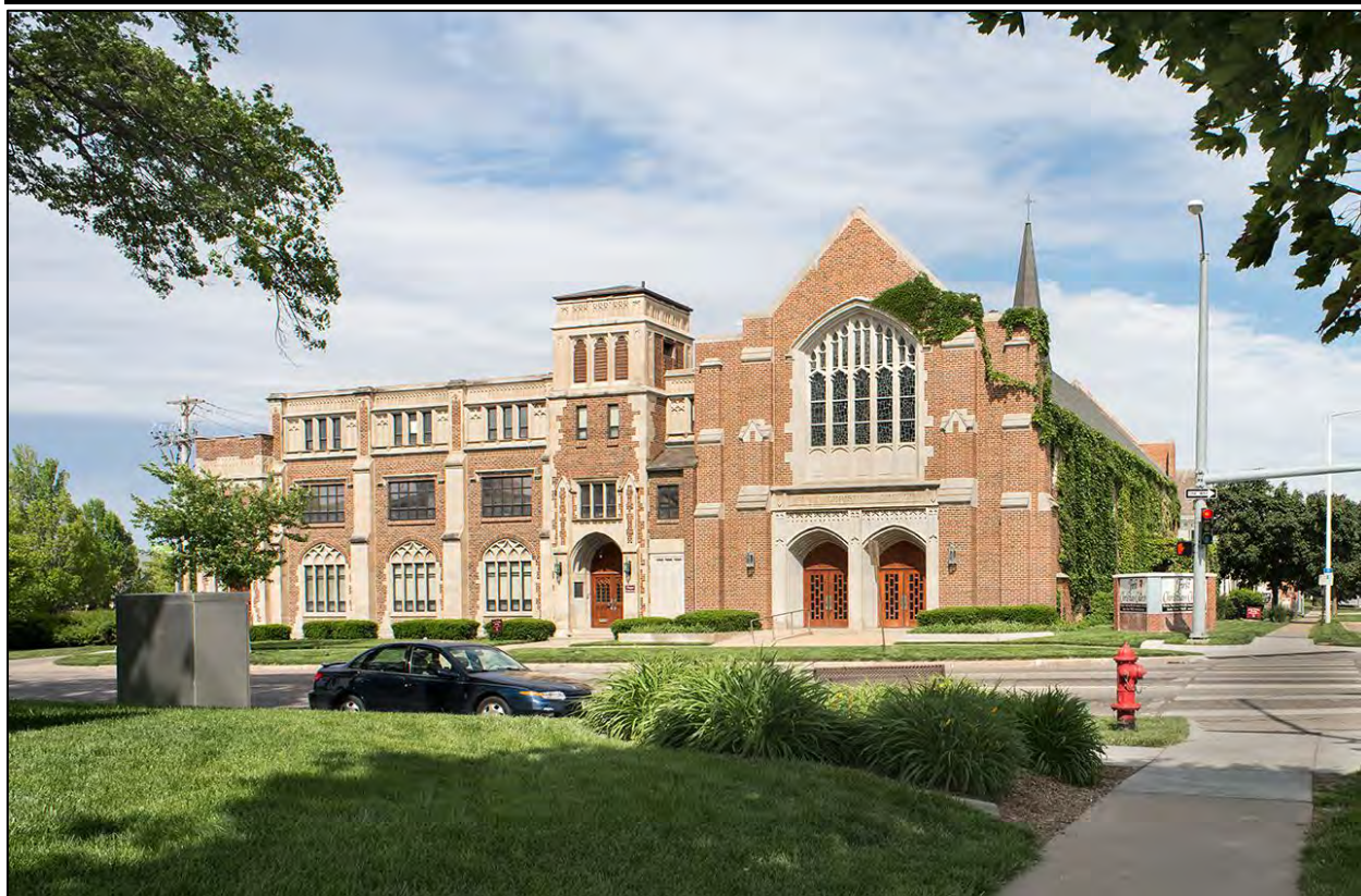
Figure 03: Façade of First Christian Church, Lincoln, NE as built 60
