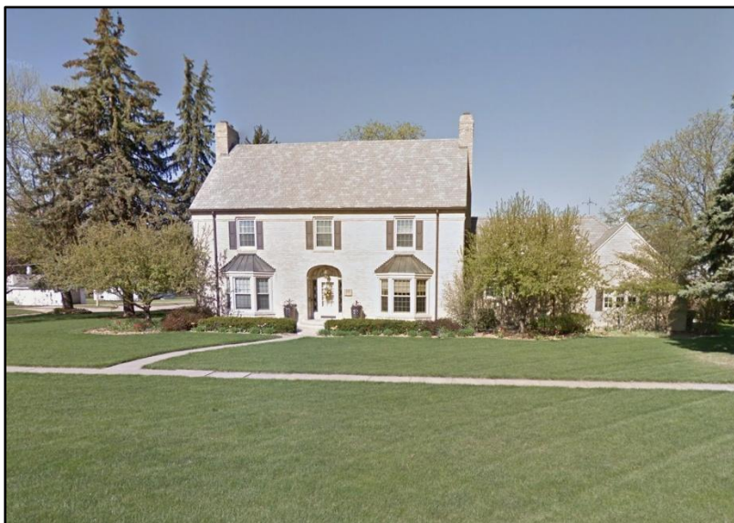
Figure 9. 823 N 4 th Street, 1938
