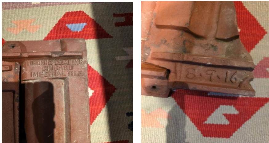
Figure 1. Photo of broken tile from roof project showing the Ludowici manufacturer mark and the manufacturer date of 8-9-1916.
