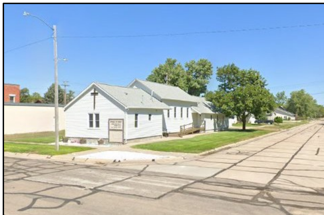
Figure 8. Church of Christ at the corner of Pine and Nebraska Streets, Ewing, NE. Google Image.
